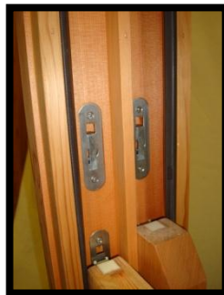
Clips Engaged for normal operation
