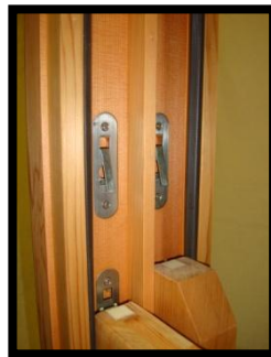
Clips disengaged for sash removal
